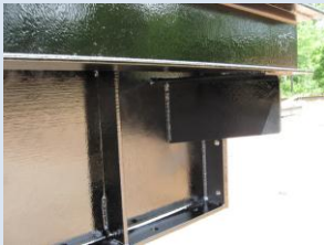
Coal tar undercoat on truck scale
