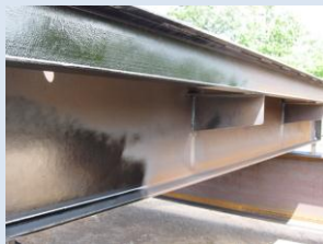
Coal tar undercoat on truck scale
