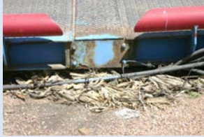
Debris beneath scale
